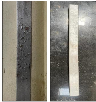
Figure 22. Buckling of column after effect of temperature
