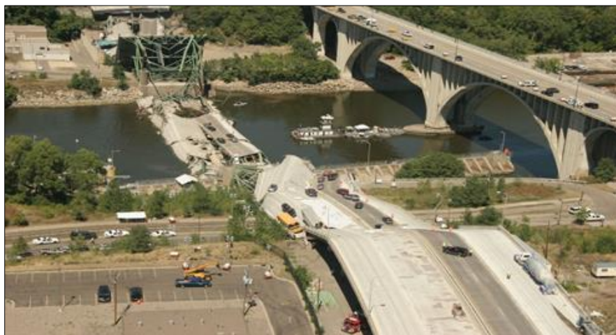
Figure 1. The failure of Mississippi (I-35W) bridge
