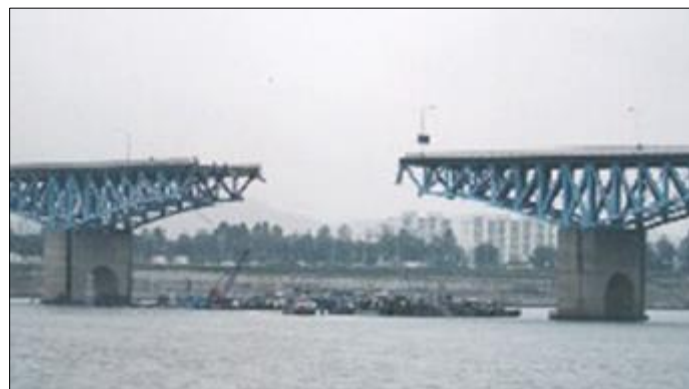
Figure 3. The failure of the bridge in Seoul despite of the local inspections [8]
