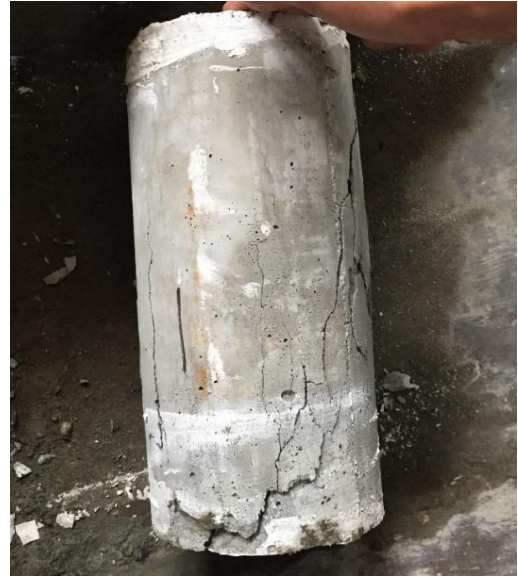
Figure 7. Cracks pattern of normal aggregate
