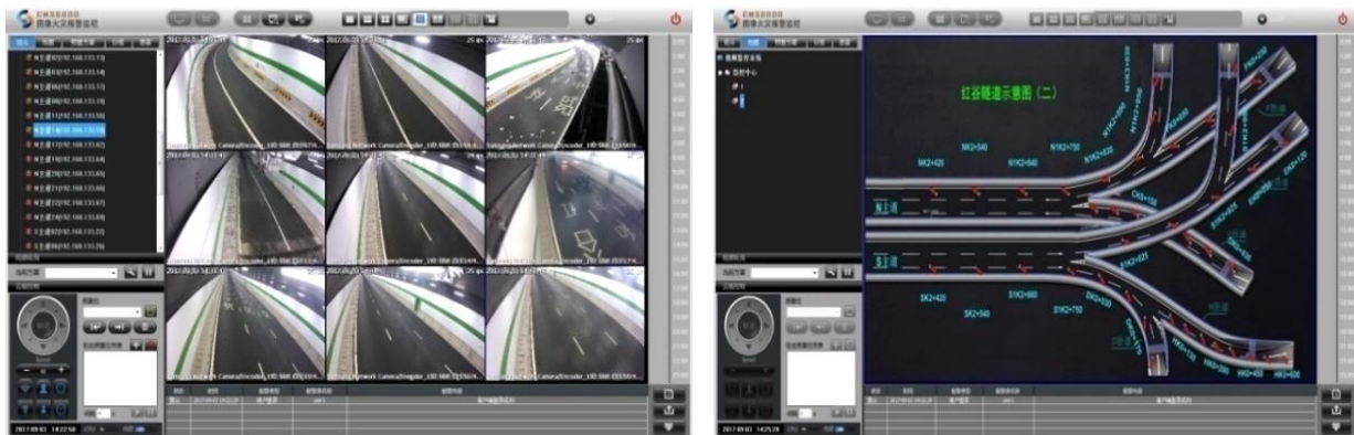
Figure 13. Display of fire VID detectors at Honggu Tunnel in Nanchang, Jiangxi
