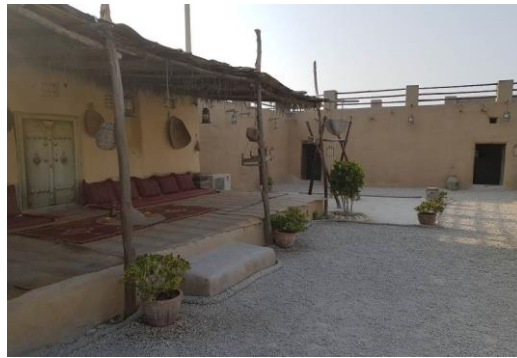
Figure 4. Using local materials to make shading space at the courtyard
