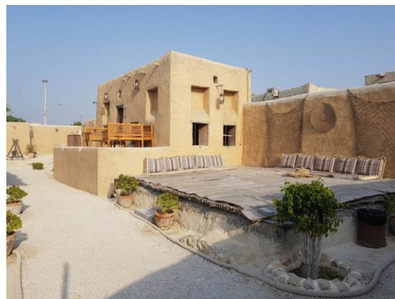
Figure 3. Using central courtyard for new public spaces for rest of visitors
