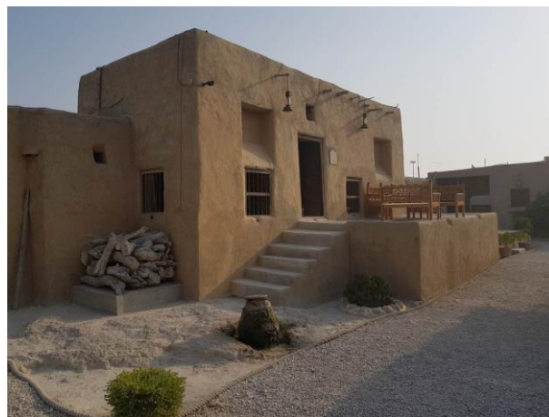
Figure 9. Using platform and different platform levels in several spaces to reduce the problems caused by ground humidity
