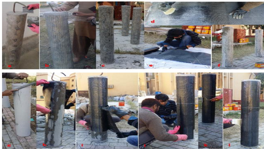
Figure 6. Repairing of Specimens
