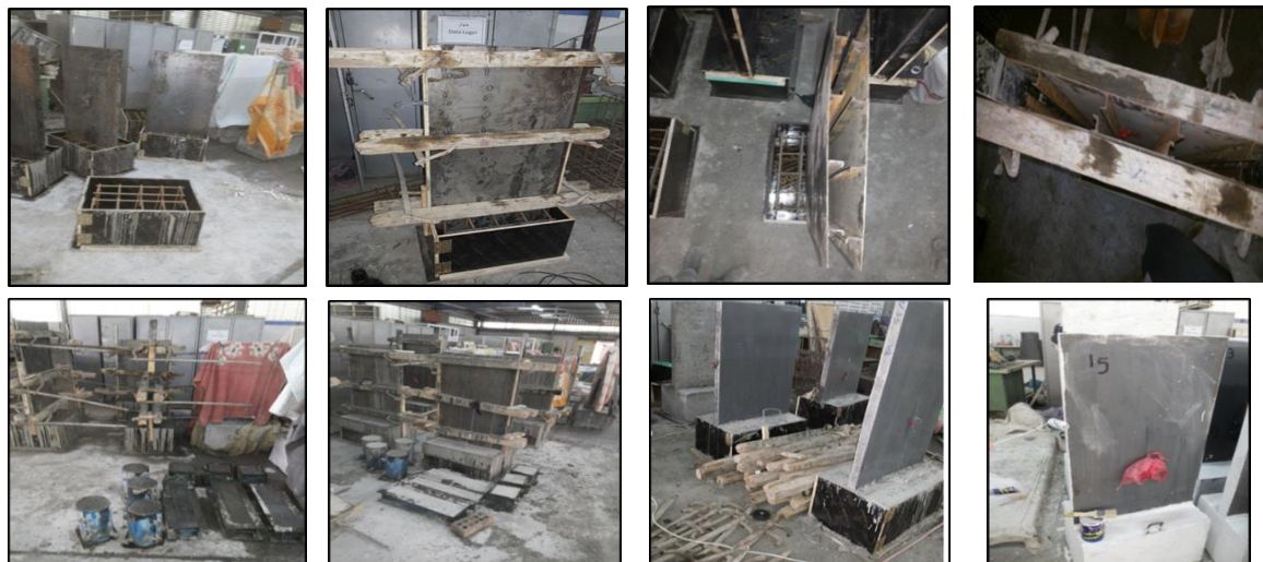
Figure 6. Casting of the walls
