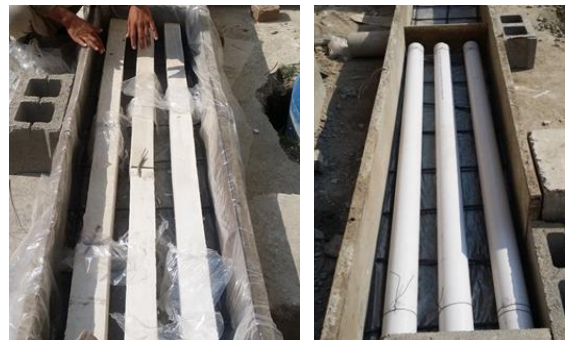
Figure 3. Casting of slab units
