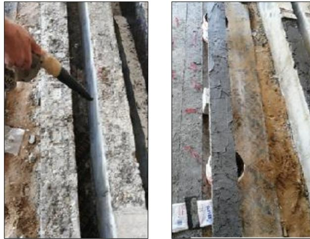
Remove and clean the concrete cover      Application of the epoxy adhesive
