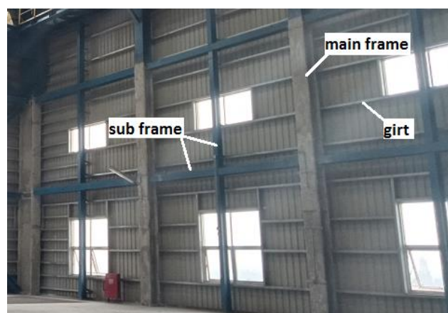
Figure 3. Reducing the span of girts by using sub-frames
