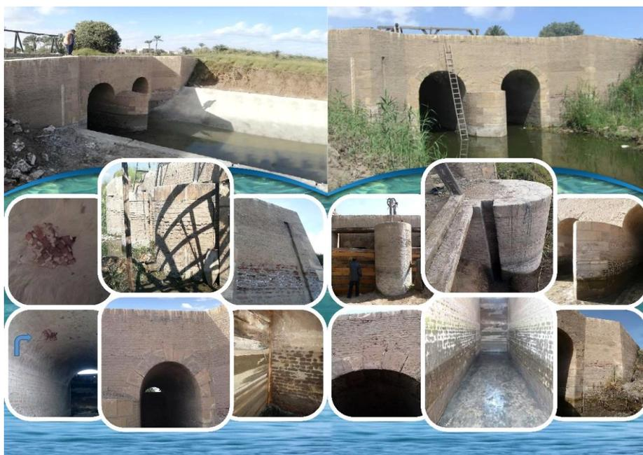
Figure 5. Visual inspection conducted to assess the apparent condition of the Regulator
