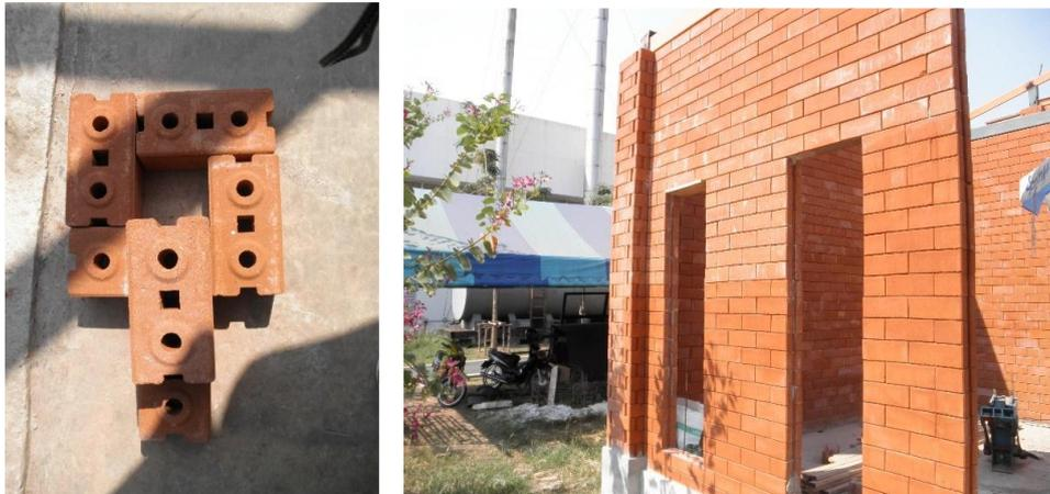
**Figure 1. Interlocking blocks and their assembly as recommended by TISTR**
