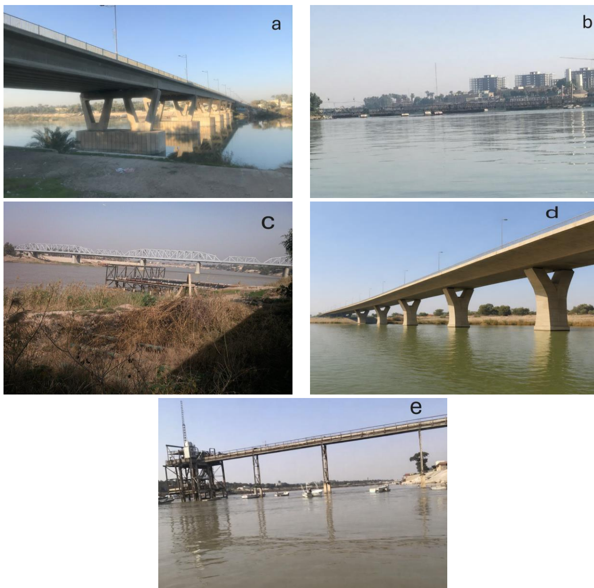
Figure 2. Images show the sites studies, a) Al-Muthanna Bridge (S 1), b) Al-Great Bridge (S 2), c) Al-Sarrafiya Bridge (S 3), d) Al-Jadriyah Bridge (S 4), e) Al-Za'franiya Area (S 5)
