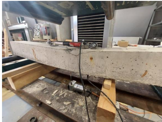
Figure 12. The failure mode of a beam in pure bending
