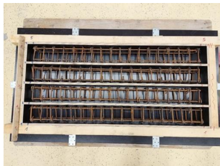
Figure 4. Formwork and reinforcement cages for the producing the beams
