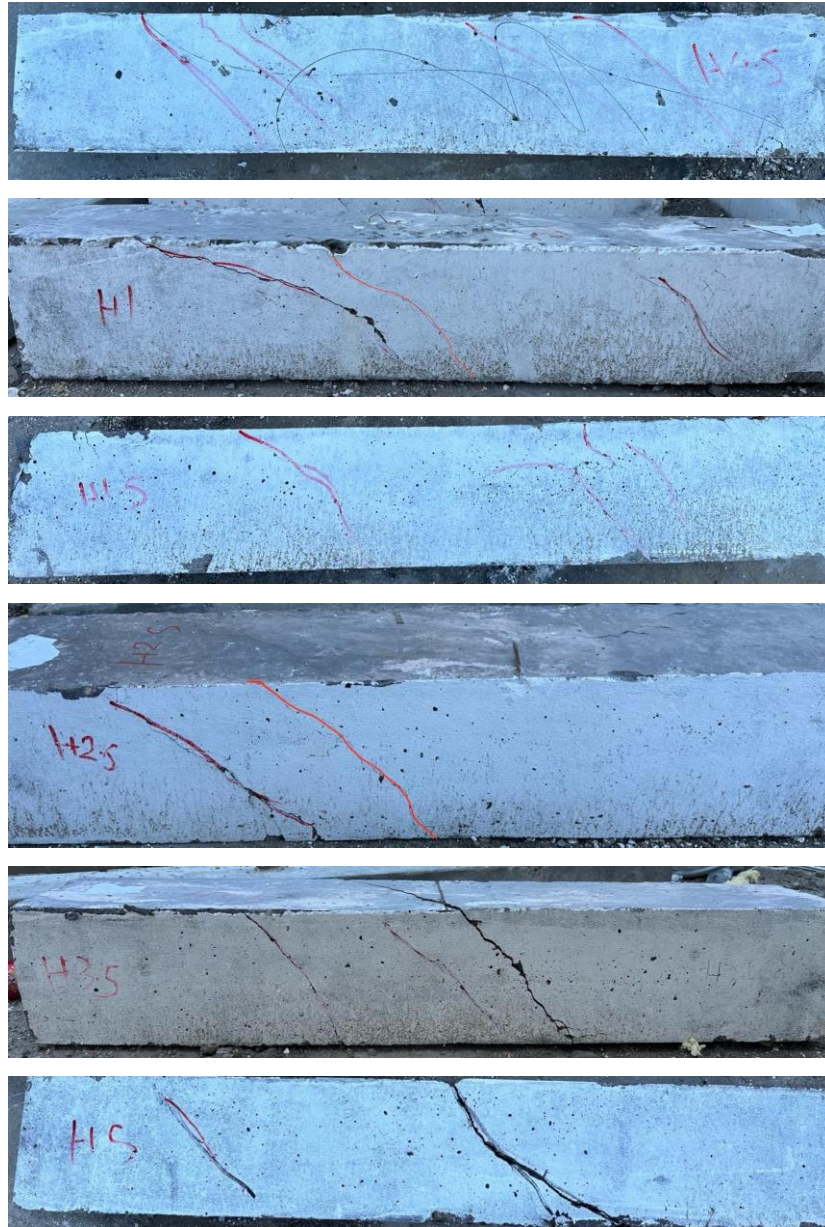
Figure 15. Failure of Second Stage Specimens
