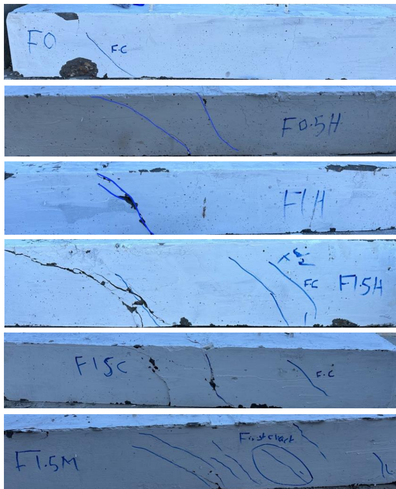
Figure 14. Failure of First Stage Specimens
