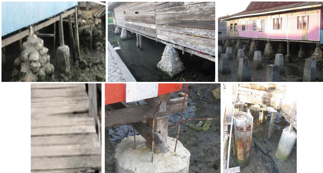
Figure 11. (a) Bajoe-Bone Settlement: Hybrid house pillars with concrete pillars at the bottom
