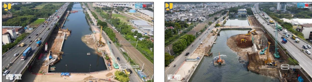
Figure 1. Project of the Sentiong Pump House, North Jakarta
