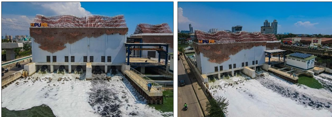
Figure 20. Pump testing after construction
