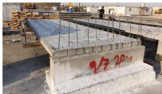
Reinforcement of rectangular and triangulate shear connectors
