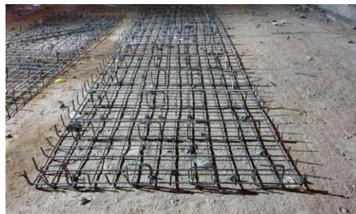
Reinforcement of pre-cast bottom layer
