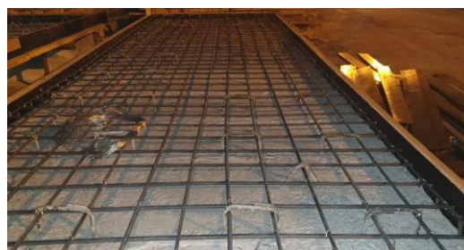
Reinforcement of cast-in-place topping layer
