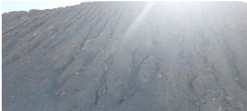
Figure 2. The clayey slope contains erosion and fracture
