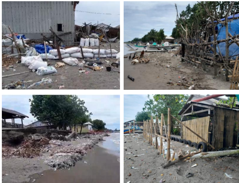
Figure 11. Types of conventional seawalls built by the community to protect their homes from wave impact and coastal erosion
