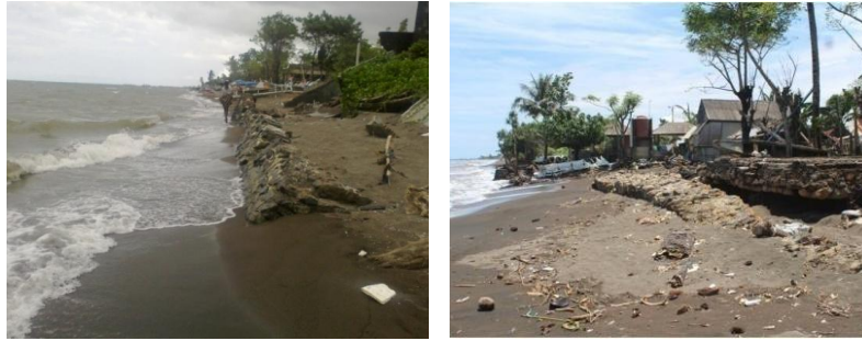
Figure 9. The Impact of Abrasion and Tidal Flooding (Rob) on Residential Construction
