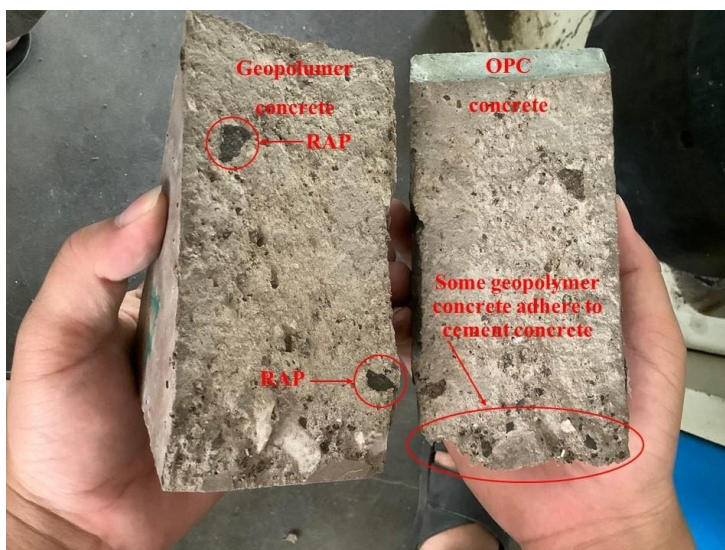
Figure 12. Characteristics of cracked surfaces between geopolymer concrete and Portland cement concrete
